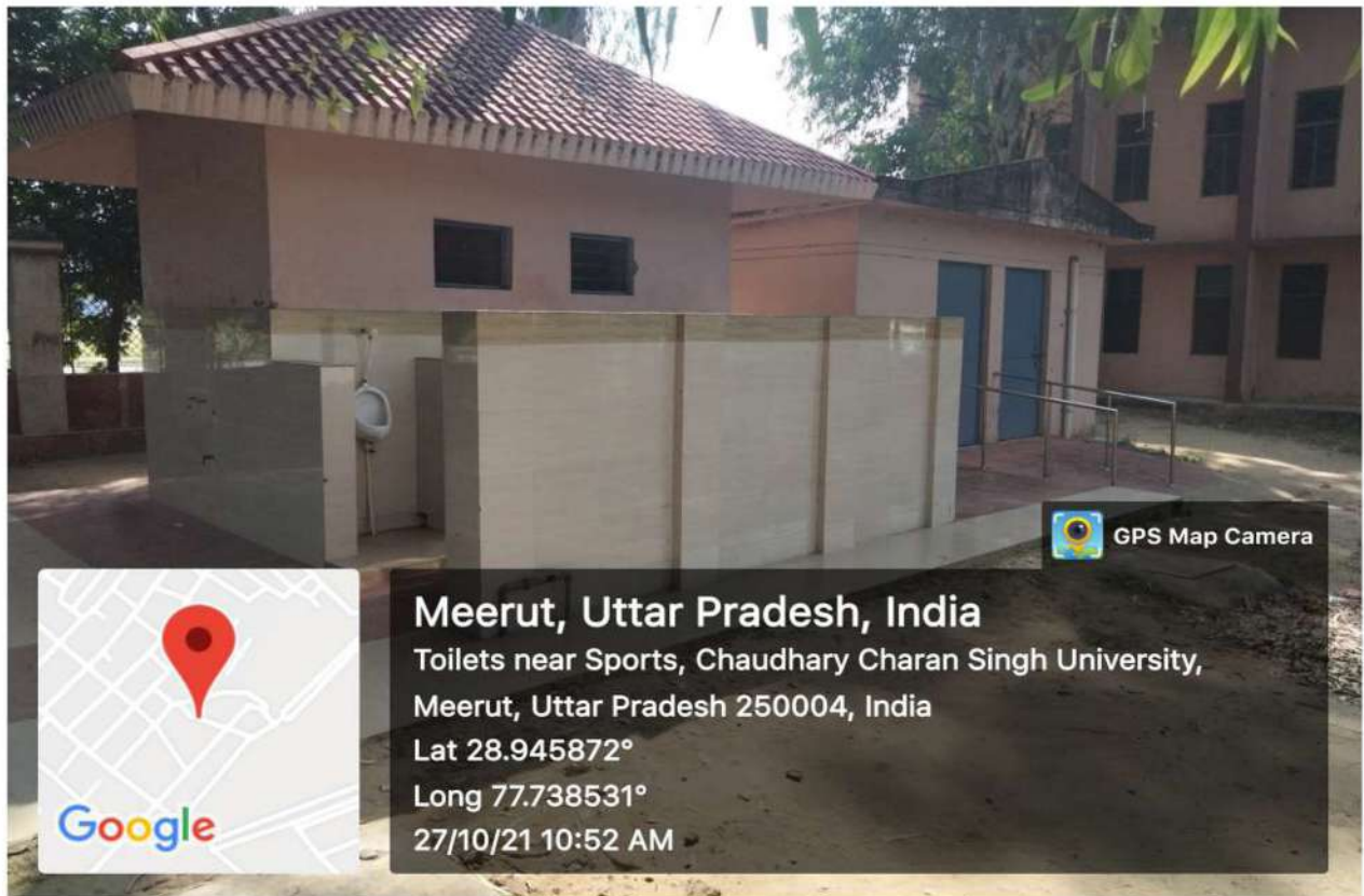
Disabled - Friendly Washroom Near Tapowan
